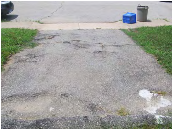
Asphalt-paved driveway surfaces exhibit age-related wear and deterioration
