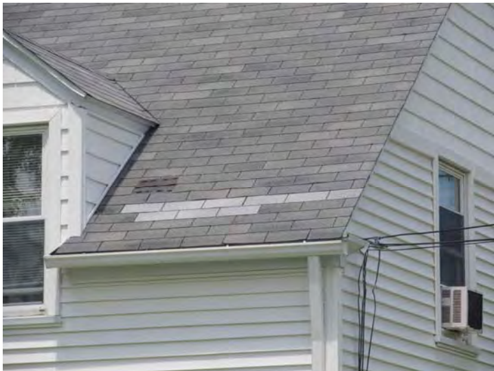
Older, three-tab, roof shingles exhibit wear and areas of past repair
