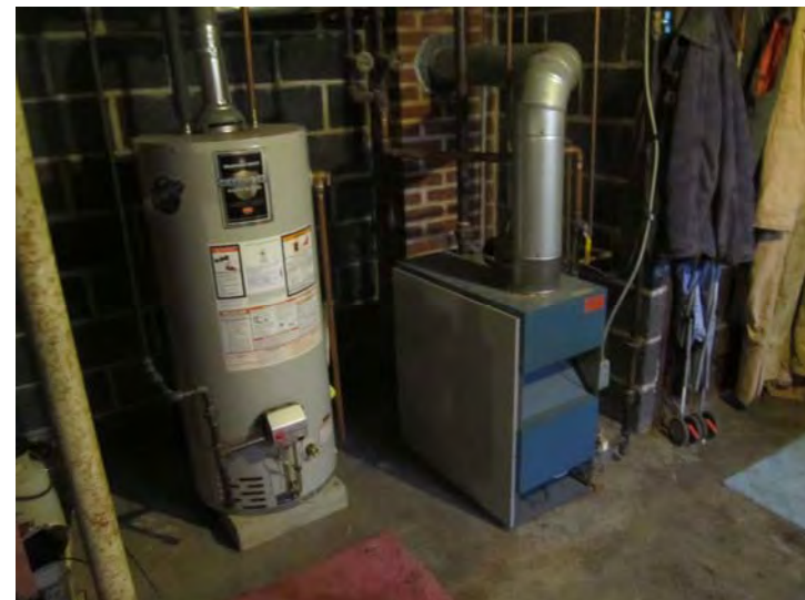
Typical, unit-level, natural gas-fired equipment for space heating and domestic hot water generation
