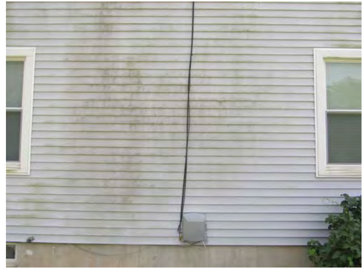
Pressure washing of vinyl to remove dirt/organic growth is needed in the near-term
