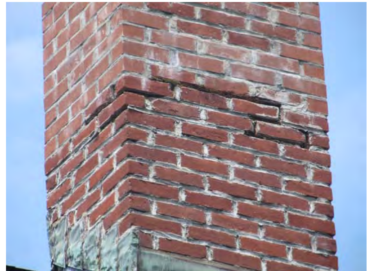
Brick chimneys in need of repair at some buildings
